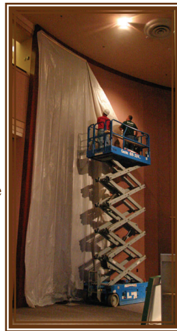
Protective sheeting has been put on the walls
