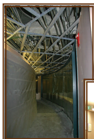
Research Area Walkway has had windows installed & bracing for new air handler equipment
